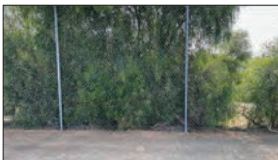
Figure 205 - Overgrowth protruding through the fence at NC Sports Complex
