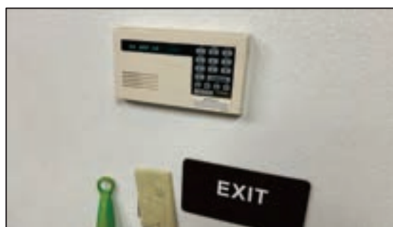
Figure 67 - Bosch Arming Station
