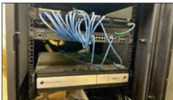
Figure 68 - American Dynamics NVR
