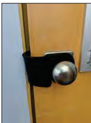
Figure 26 - Lock Blok Strap
