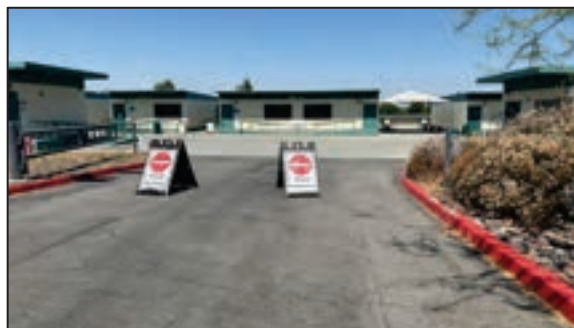
Figure 146 - Unsecured Swing Arm Barrier (MVC Portables)
