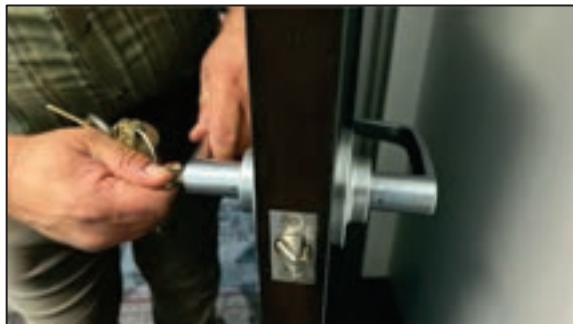
Figure 96 - Cylindrical lockset with no internal locking option – SSV Building (NC)
