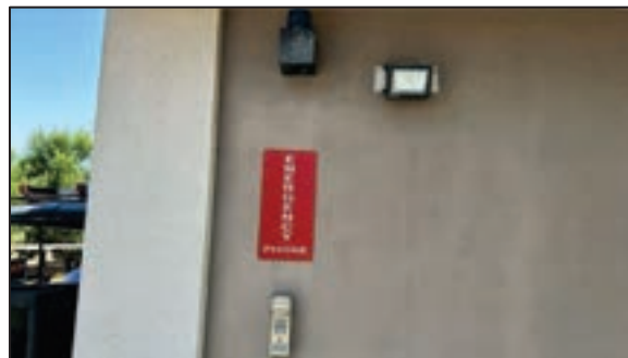
Figure 326 - Trigon Wall Mount Call Station w/ Independent Blue Strobe
