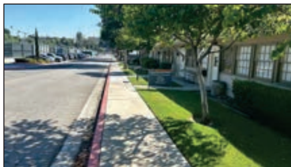
Figure 12 - RCC Facilities Building
