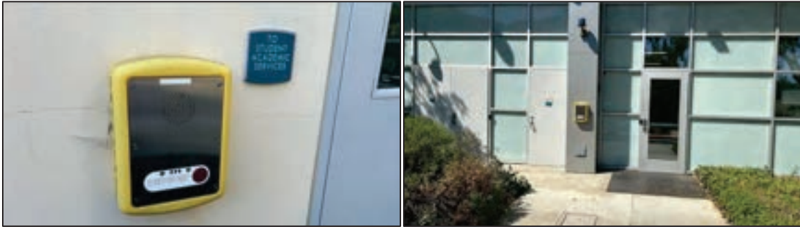
Figure 304 - Code Blue Wall Mount Call Stations w/ Independent Blue Strobe
