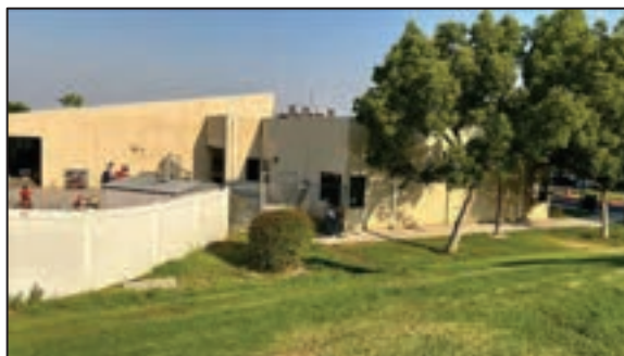
Figure 183 - Fencing and Gates at ECEC MVC Playground
