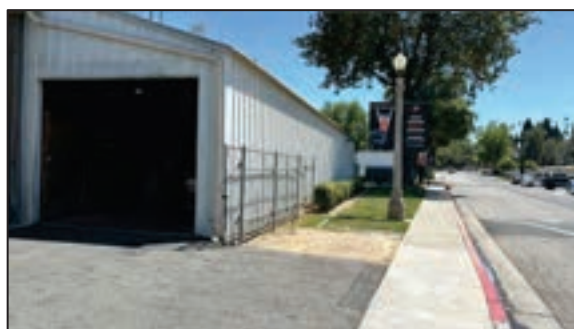
Figure 157 - Speed bump (RCC Warehouse)
