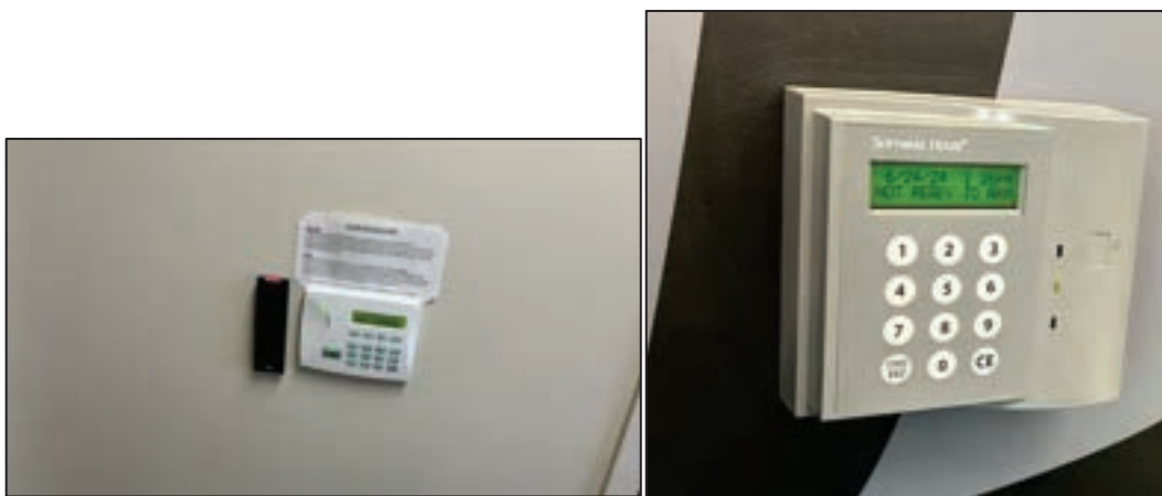
Figure 66 - MVC Intrusion Arming Station w/ Card Reader and Software House RM Card Reader
