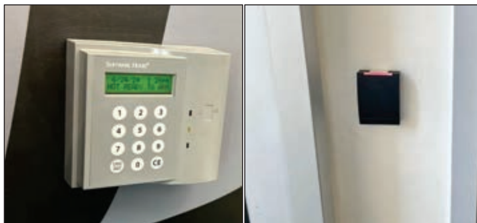
Figure 60 - Software House RM Card Reader Keypad and Siemens (HID) RP40 Card Reader
