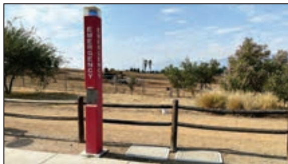
Figure 41 - Wooden lodge pole rail fence line with rotting posts at NC
