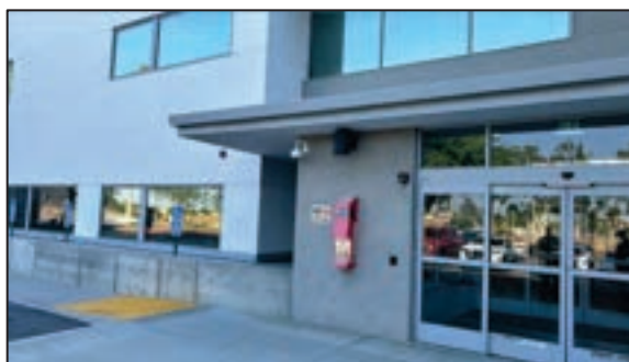
Figure 27 - NC CSS Building
